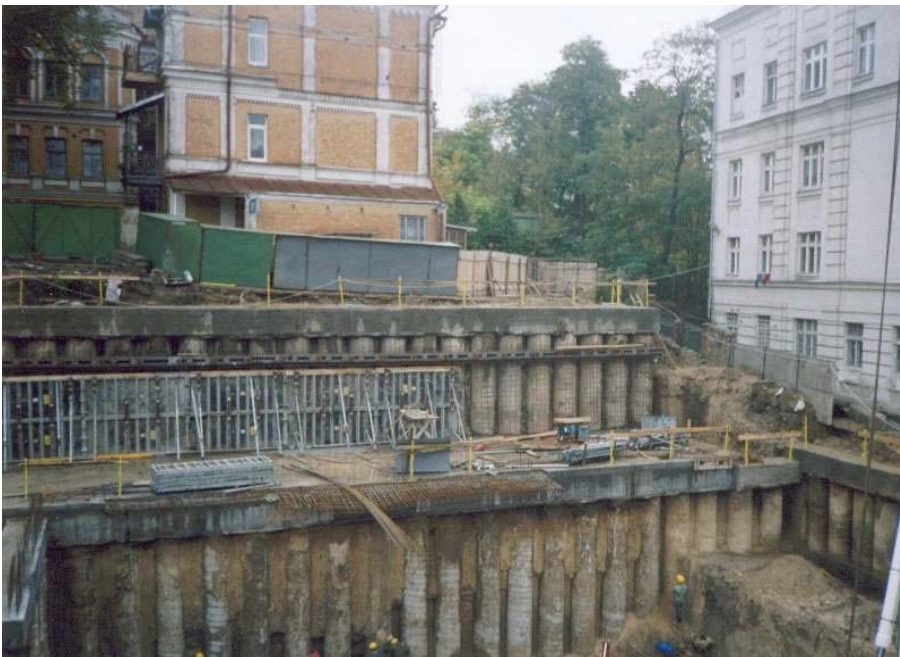
Fig.4. An example of the deep excavation for the new construction in the conditions of dense buildings and complex geological conditions in the Pechersk district of the Kyiv city. Source: the author's photo
