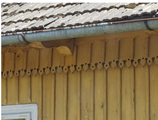
Fig. 6. Profiled eaves beam, decorated boards on the façade, vertical arrangement of boards, house in Zagorzyce near Ropczyce; Subcarpathia, Poland; Source: author's photo
